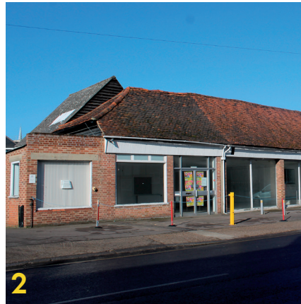
2 Dane St corner
