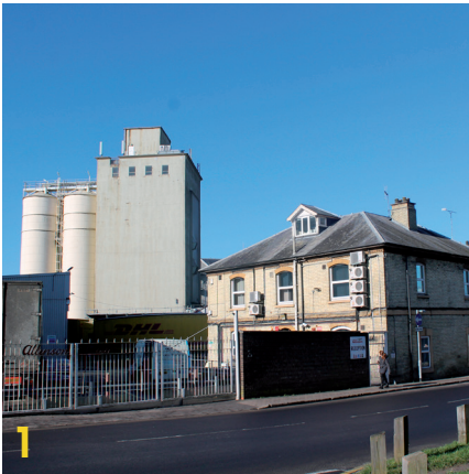
1 Flour Mill from Dane Street
